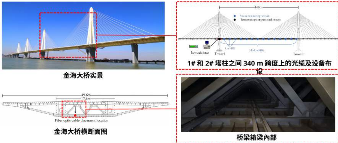
Figure 2. Target monitoring area: the 340 m span between Tower 1 and Tower 2, including cross-section and cable placement region inside the box girder.
